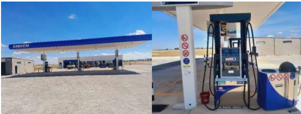
Figure 2-1: The canopy and fuel pumps island onsite
