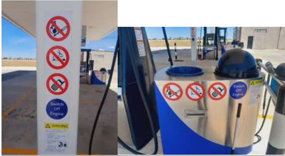
Figure 2-11: Some of the warning and prohibition signs at the fuel pump island onsite
