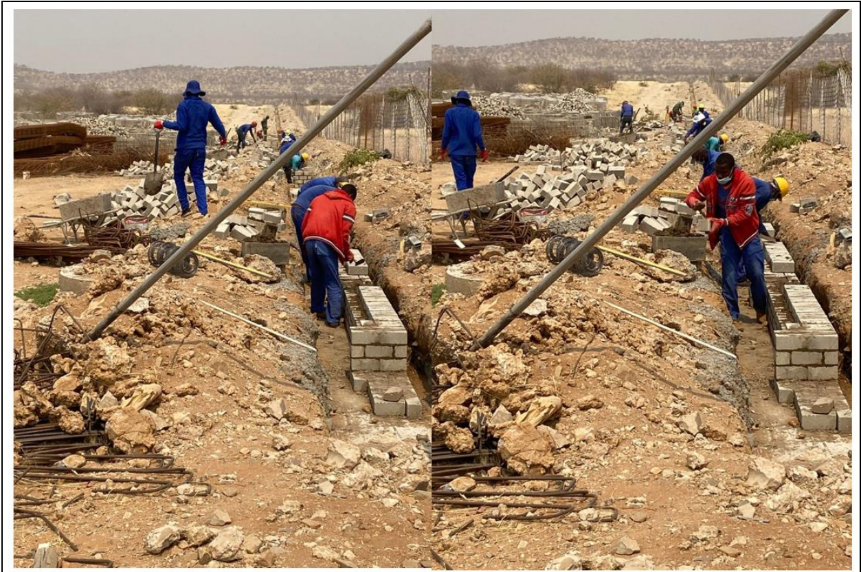
Figure 5: Construction of the boundary wall between the workshops and cemetery
