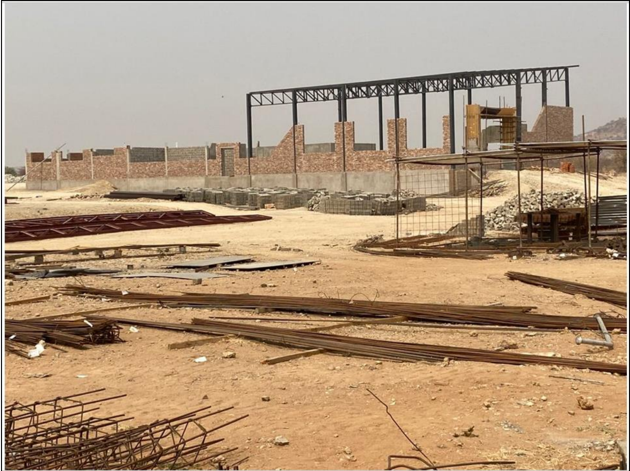
Figure 7: Workshops foundations and steel structure
