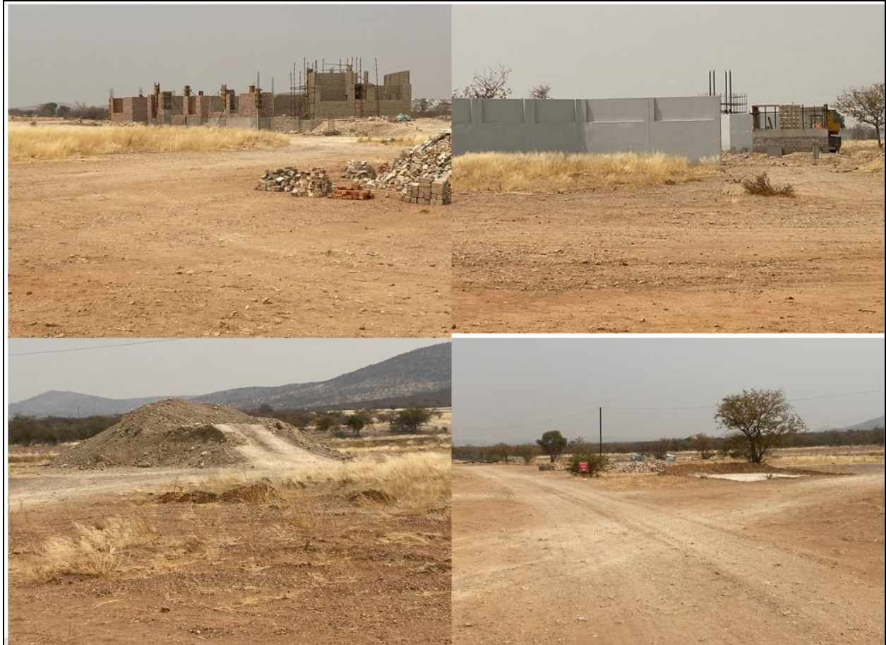
Figure 9: Stockpiling of the soil and overburden materials for backfilling during construction and rehabilitation
