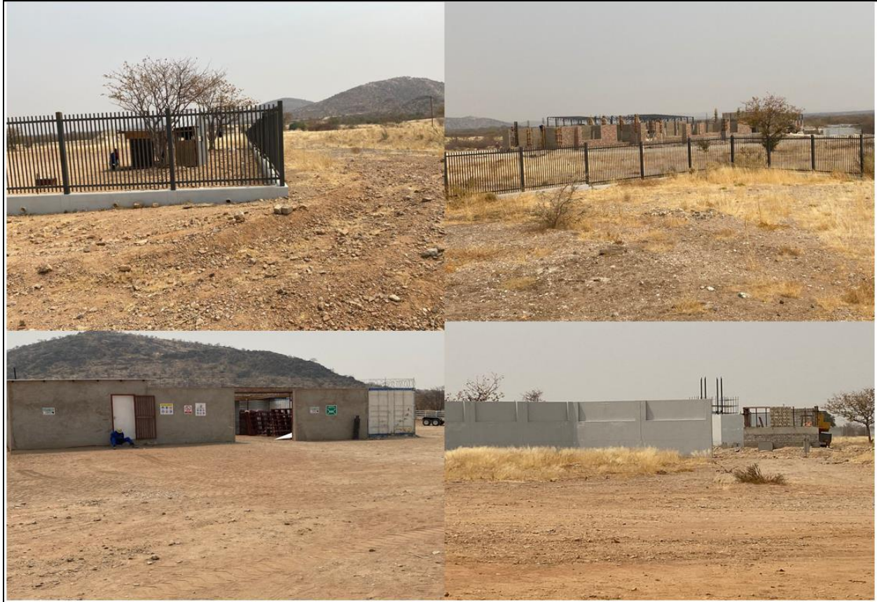
Figure 8: Boundary wall, contractor site office, and guardroom
