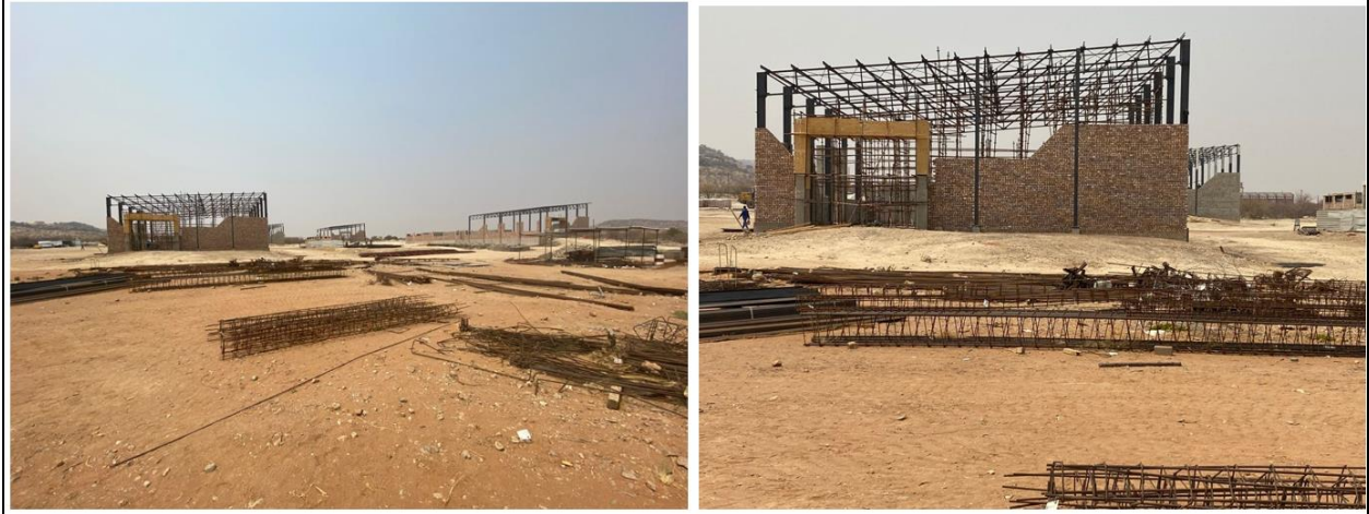
Figure 4: Workshops construction progress
