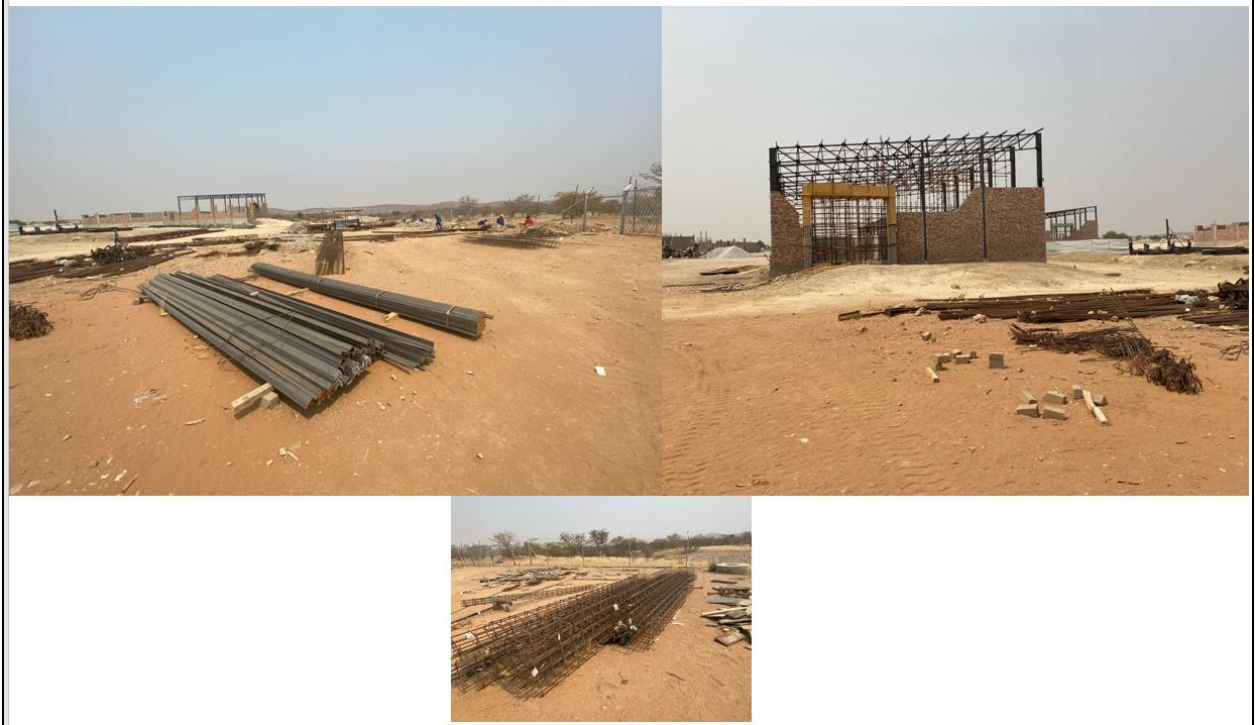
Figure 6: Onsite steel construction materials and workshops structure
