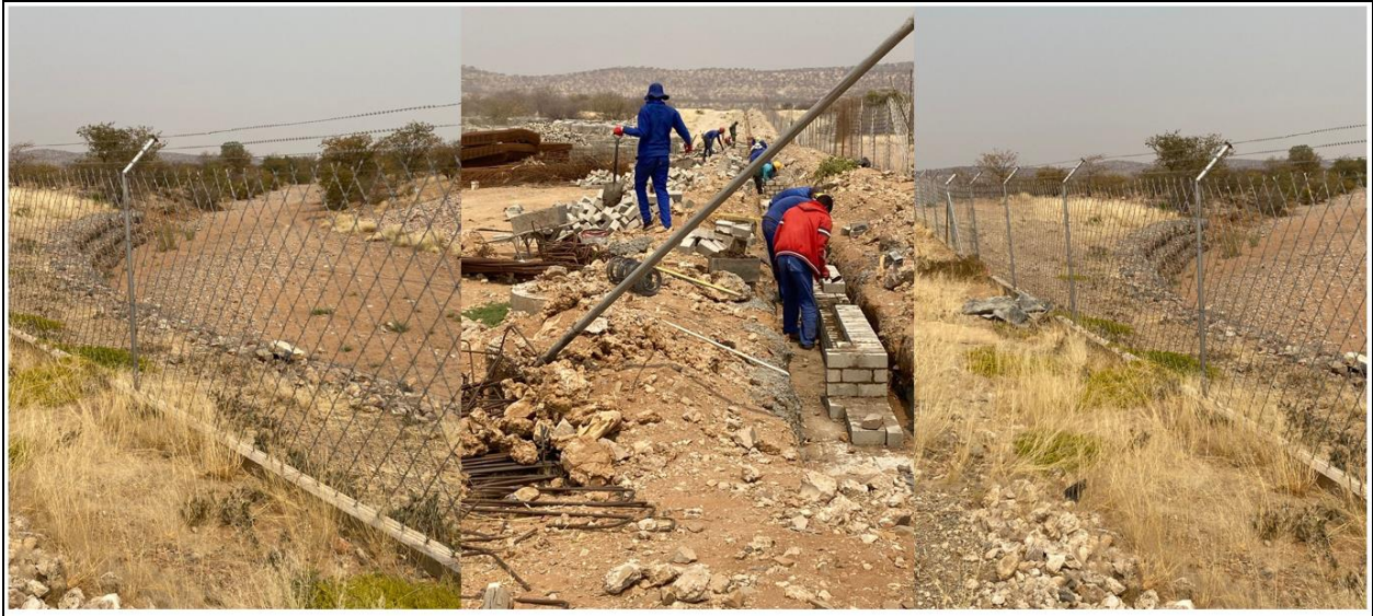
Figure 10: Installation of gabion wire and boundary wall
