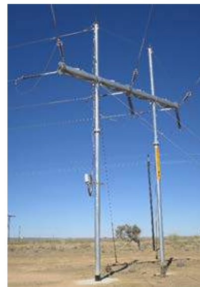
Photo 4.5.3 - View of H-structure pole design (to be stayed)
