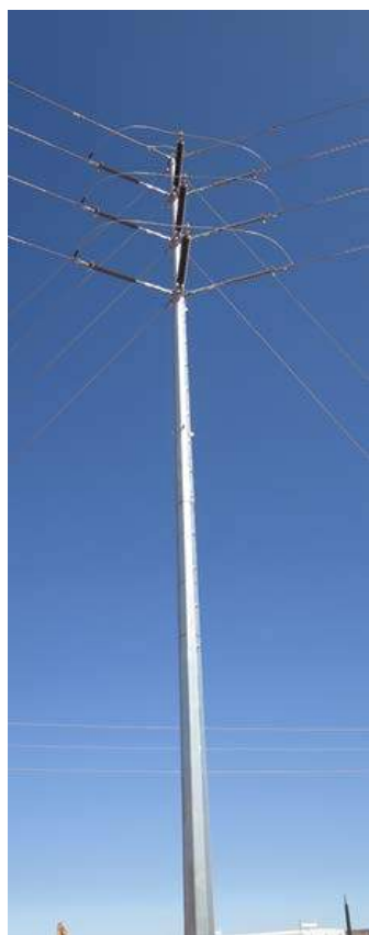
Photo 4.5.2 - View of single-circuit angle steel monopole structures (to be stayed)
