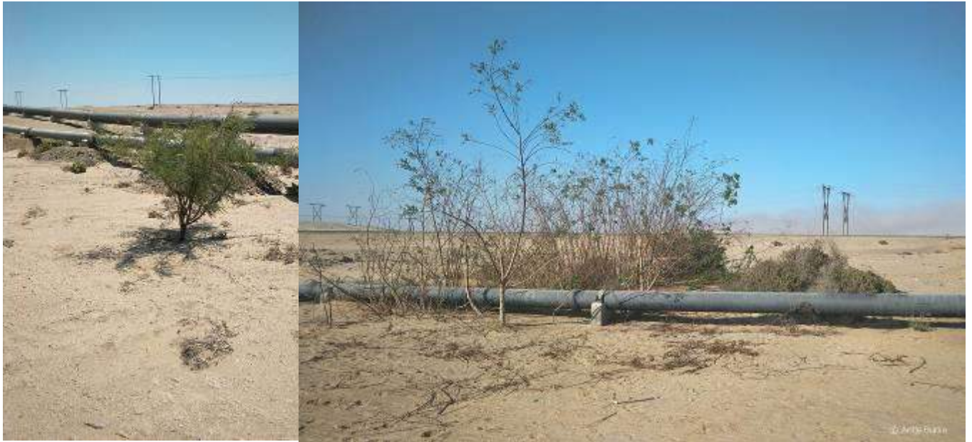
Figure 12. Invasive alien plants spring up where there are leaks along the pipeline – here a mesquite ( Prosopis species) at left and wild tobacco ( Nicotiana glauca ) on the right.
