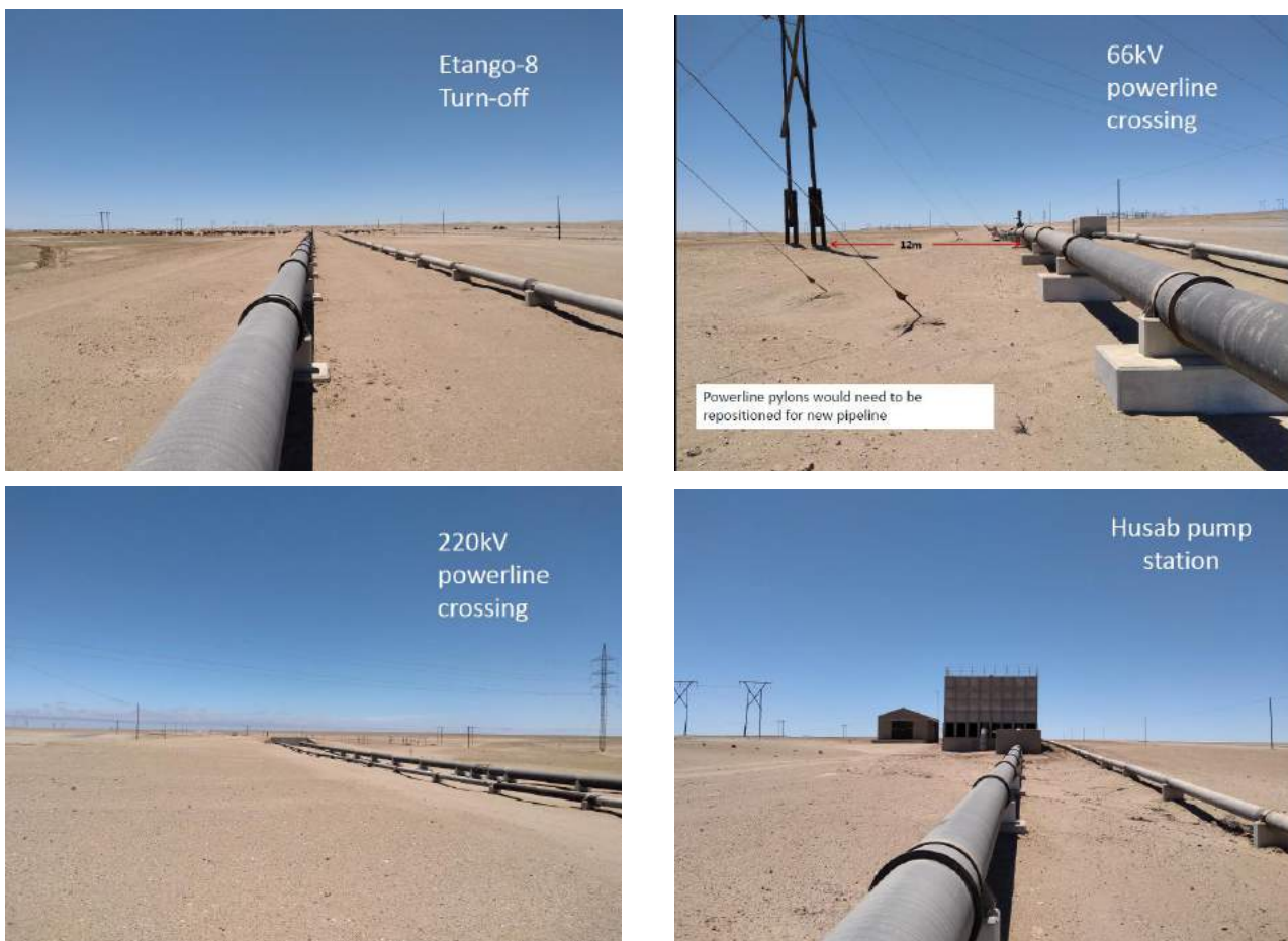
Figure 4: Existing infrastructure corridor, which will also accommodate the new Etango Project water pipeline.
