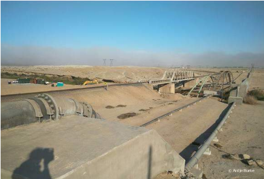
Figure 5. Existing pipelines crossing the Swakop River.
