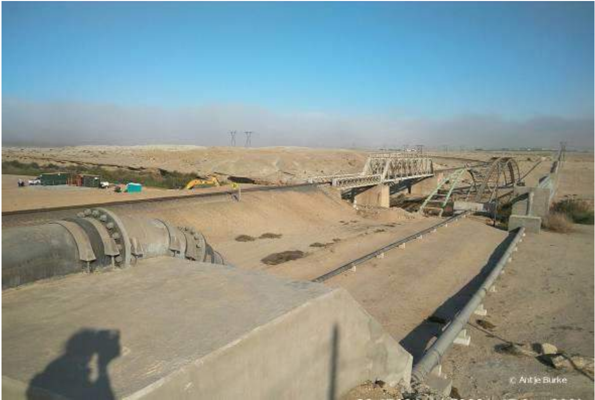
Figure 5. Existing pipelines crossing the Swakop River.
