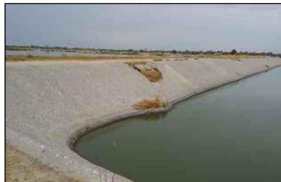
Figure 12: Oshakati East Ponds – Minor damage to embankments
