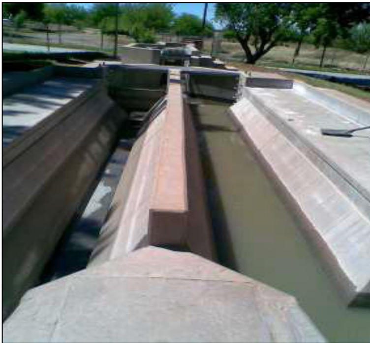
Figure 18: Proposed inlet works with grit removal channel
