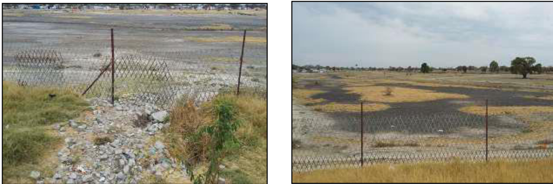
Figure 14: Oshakati East Ponds – Final water health hazards at the ponds
