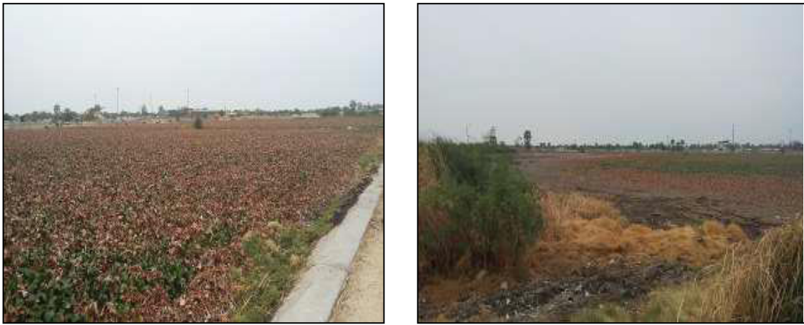
Figure 5: Oshakati West Ponds – Primary ponds overgrown
