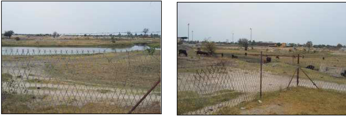
Figure 7: Oshakati West Ponds – Final water discharge outside pond areas
