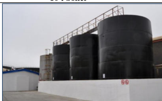
Photo 2-4 Fish oil storage tanks
