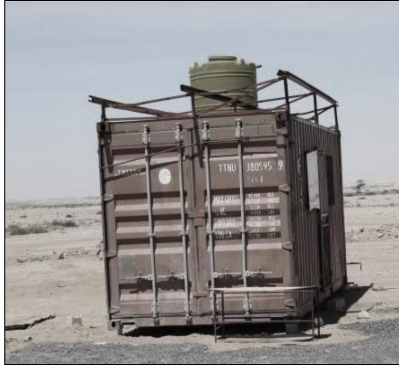
Figure 2-1. Typical containerized ablution and sanitation facility to be erected on site
