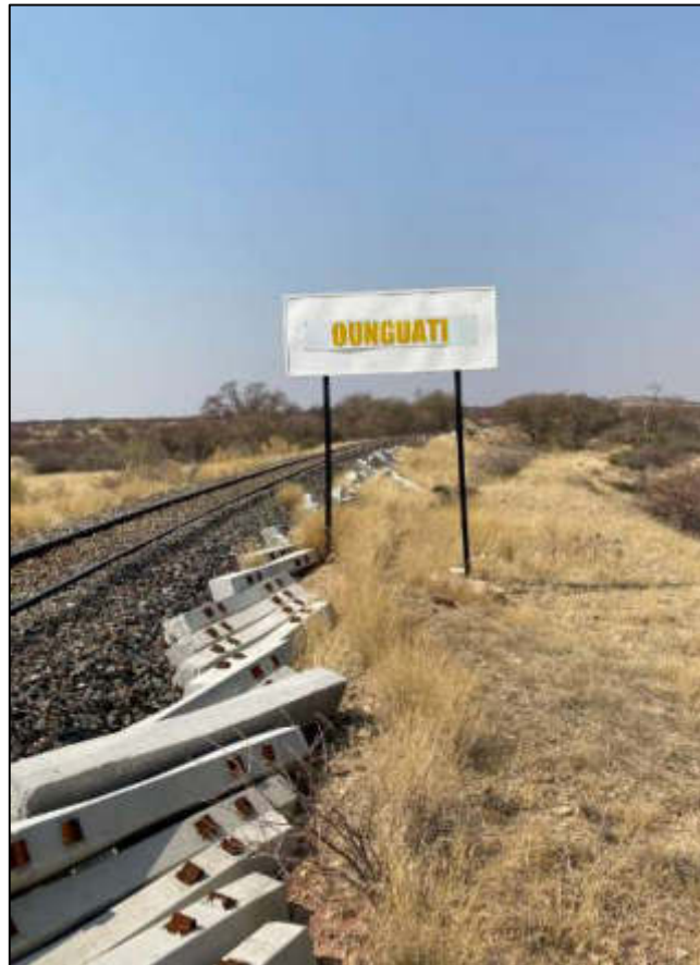
Figure 4-10: Kranzberg Railway Line located south of MC 72499 - 72503.
