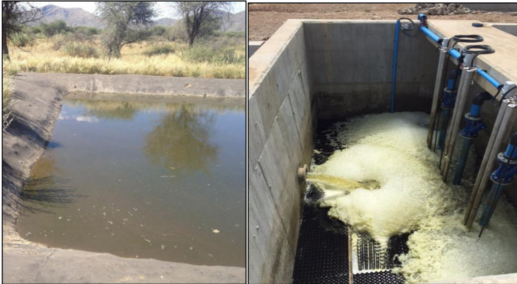
Figure 13: Treatment of effluent
