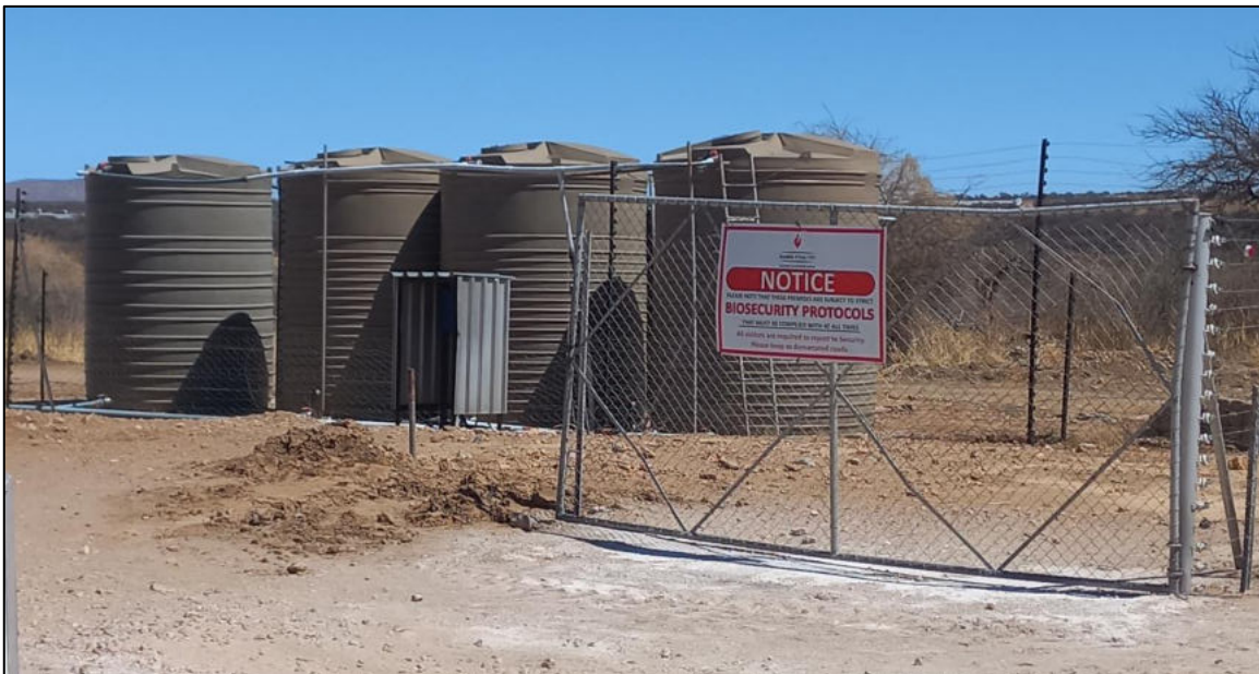
Figure 10: Water tanks on site
