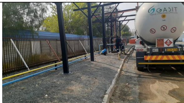
Photo 3. Gantry for offloading LPG
