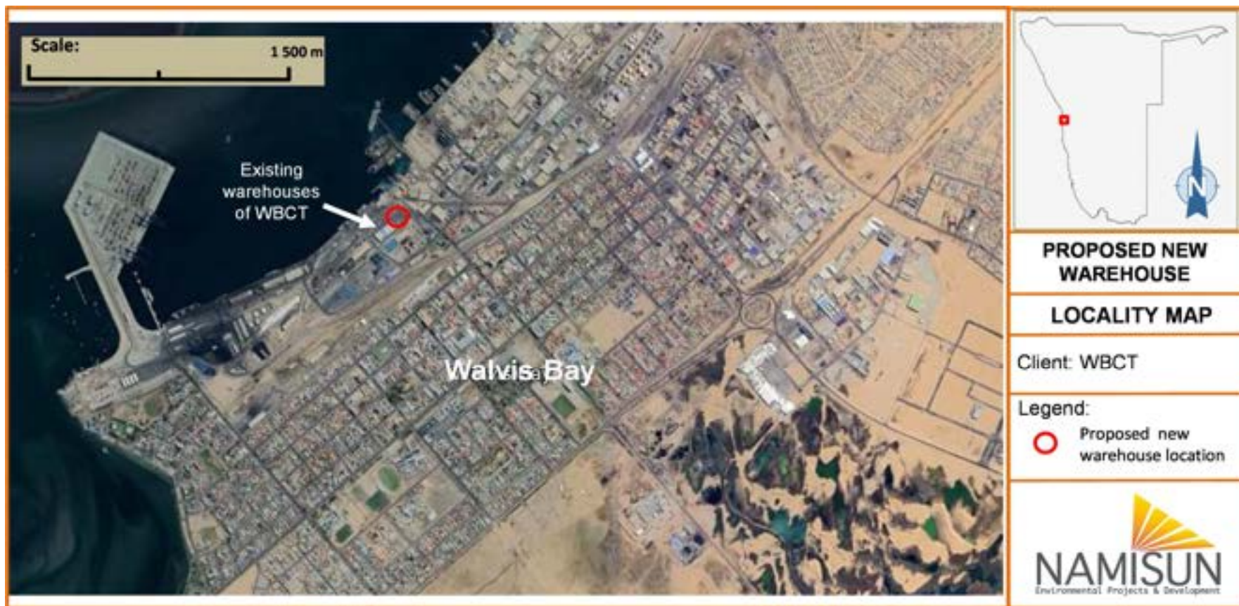
FIGURE 1: LOCATION OF THE PROPOSED NEW WAREHOUSE, RELATIVE TO THE EXISTING FACILITIES ON THE WBCT SITE IN THE PORT OF WALVIS BAY
