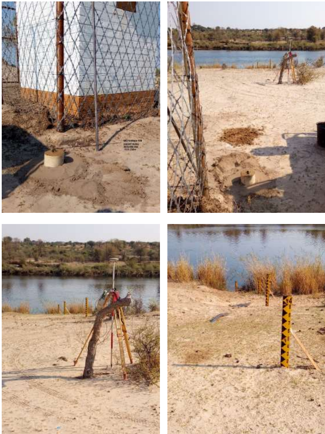
Figure 3 Existing hydro-gauging infrastructure
