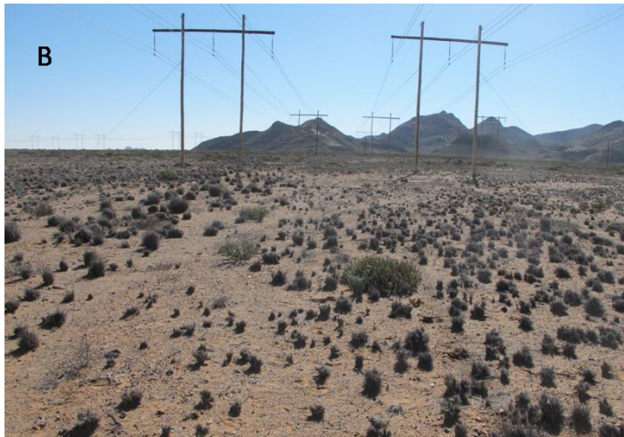
Plate 2: The corridor of damage along the existing power line north of the Obib substation, showing very low re-establishment of succulent and perennial plant diversity. A = undamaged; B = damaged.
