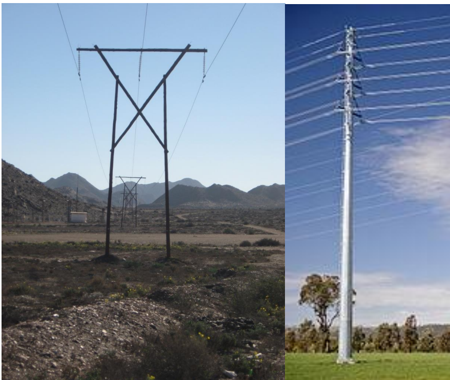
Plate 1: Example of twin pelican conductors and single pelican conductors.
