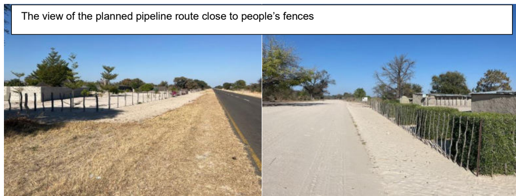
Figure 4: The overview of the visited project route with private properties along or falling within the planned pipeline around the Siyoka and Silumbi areas
