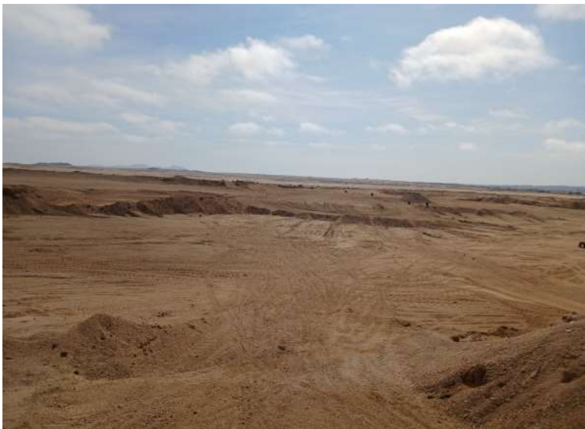
Picture 3 Borrow pits showing clear and abundant G5 material.
