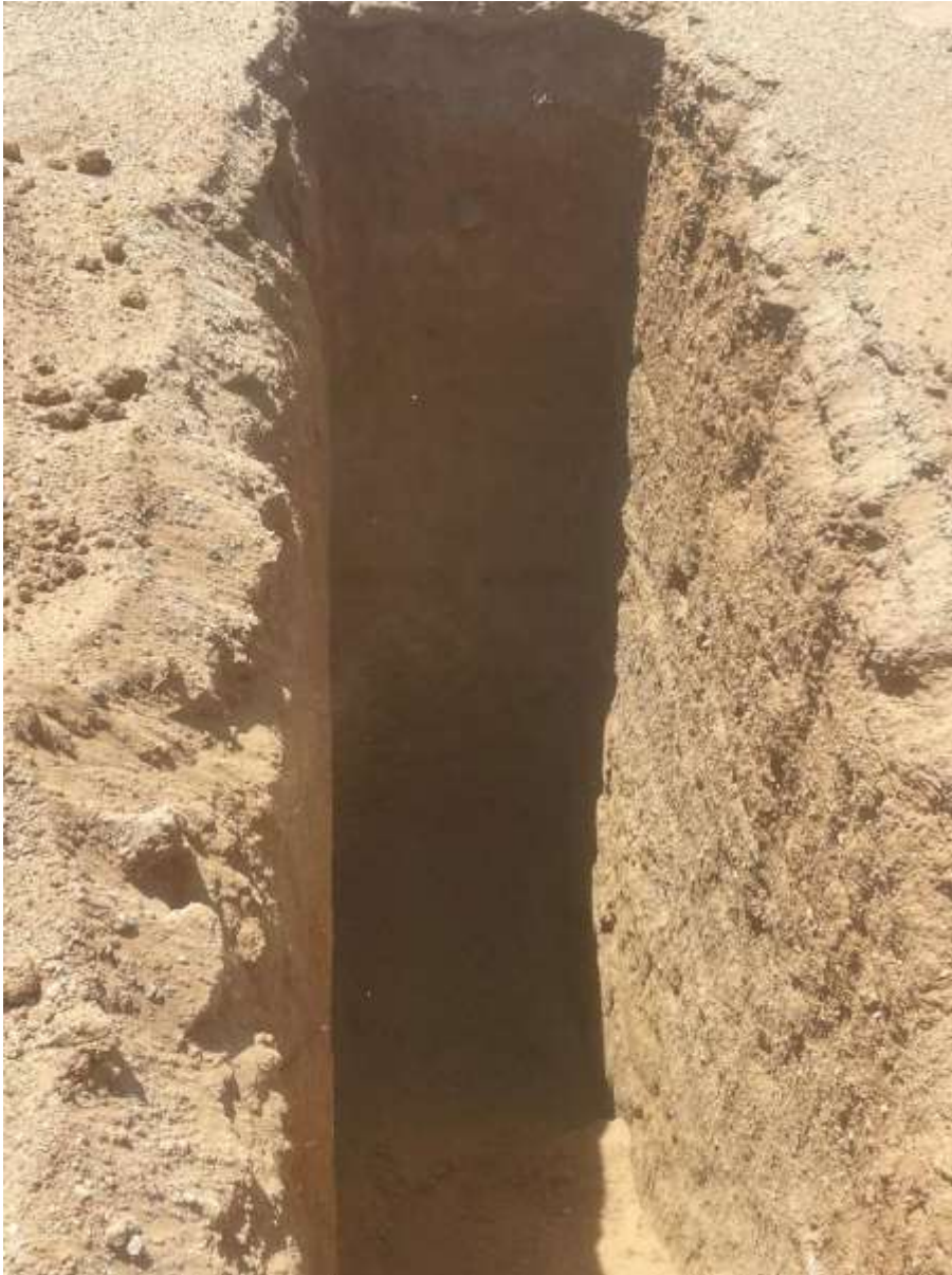
Photo 5: TEST PIT NO.2
