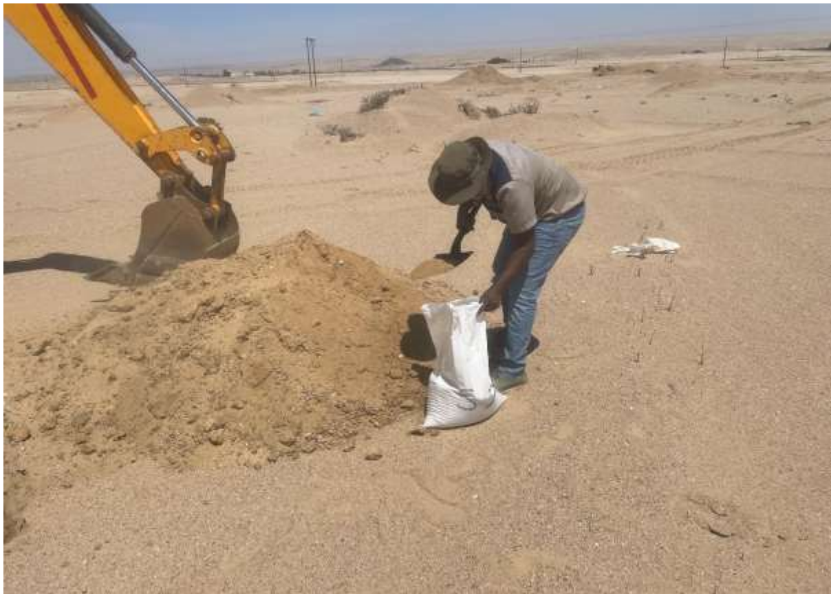
Photo 3: TEST PIT NO.1
