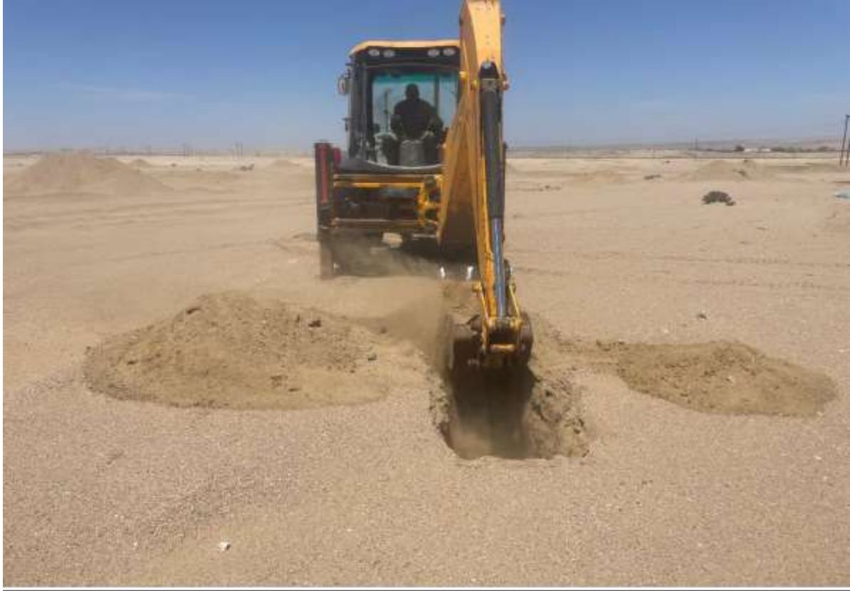
Photo 2: TEST PIT NO.1
