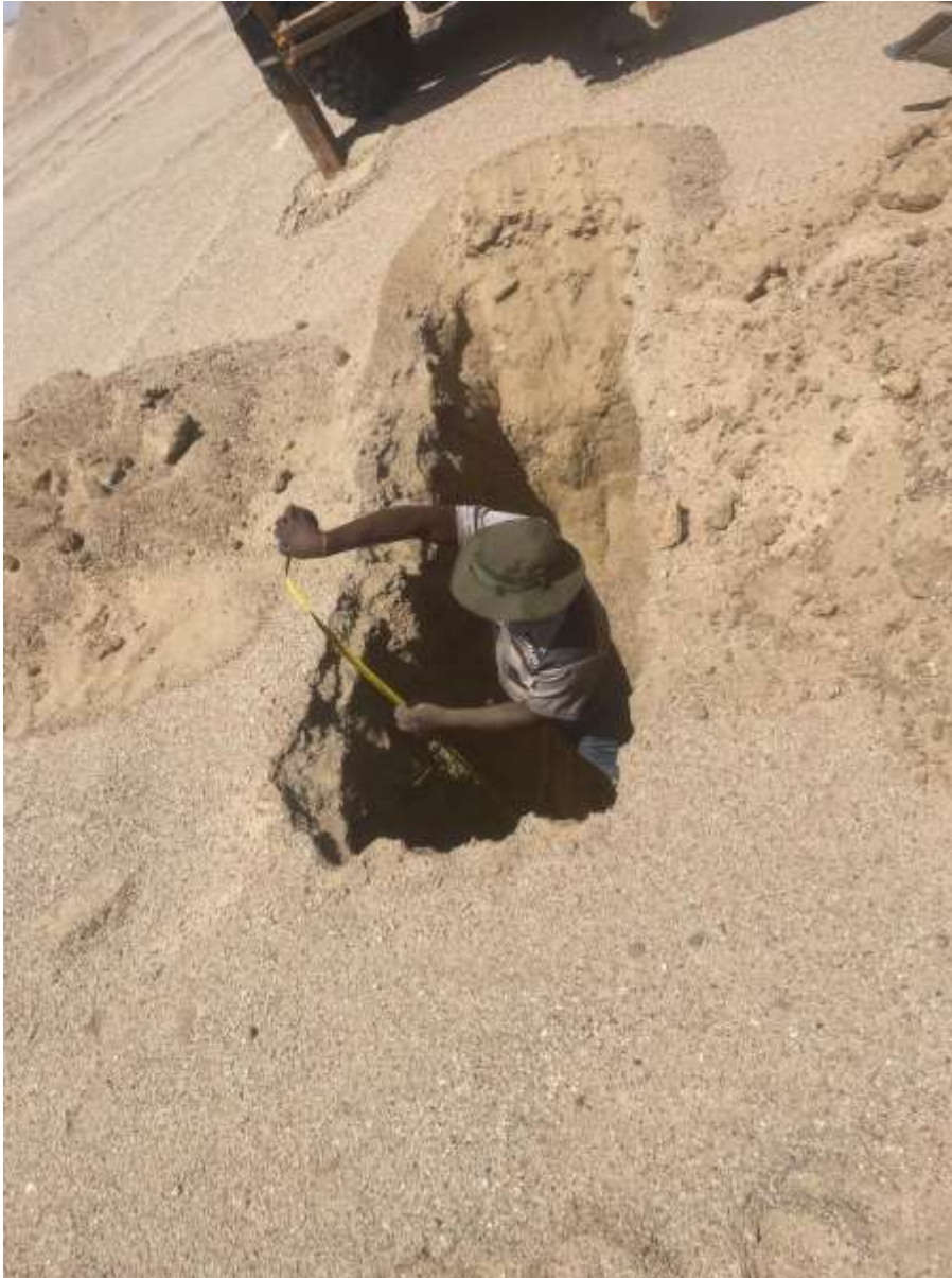
Photo 4: TEST PIT NO.2
