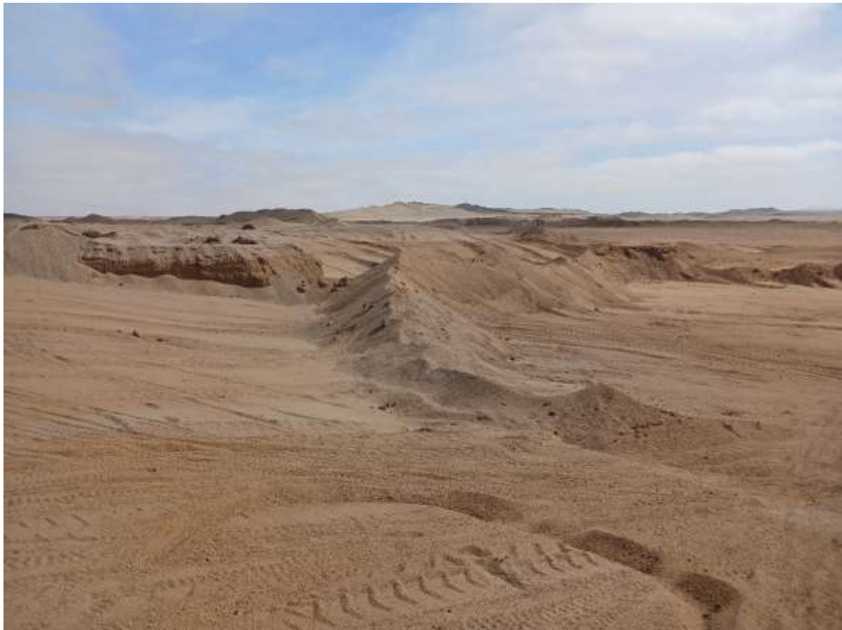
Picture 4 Active borrow pit excavated to G5 material.
