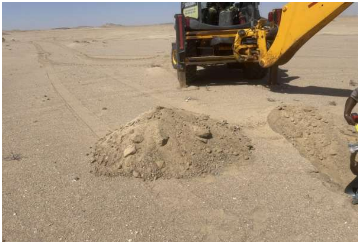
Photo 8: TEST PIT NO.5
