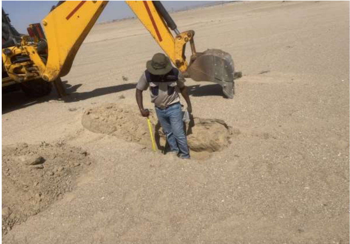
Photo 7: TEST PIT NO.4
