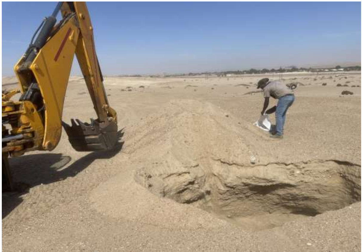
Photo 12: TEST PIT NO.9
