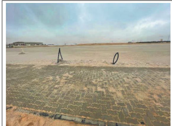
Photo 4-2 Utilities installed on site
