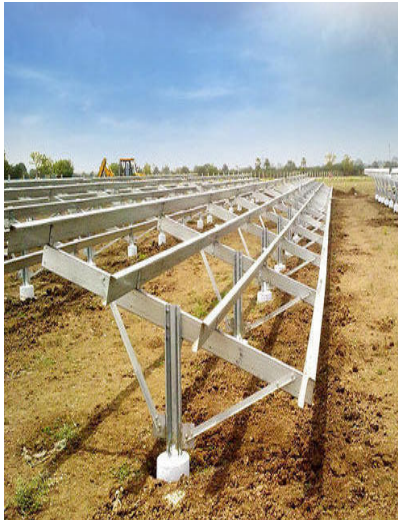
Figure 4: Completed PV Panel Mounting
