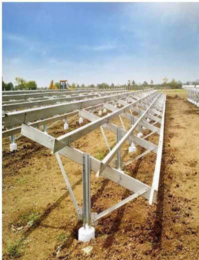
Figure 3: Completed PV Panel Mounting
