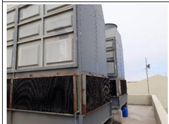
Photo 4-28 Evaporative coolers
