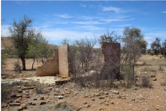
Figure 19: Ruins of old building structures (Source: Author, 2024)
