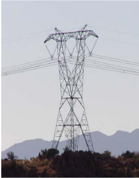
Figure 4: Self Supporting Tower
