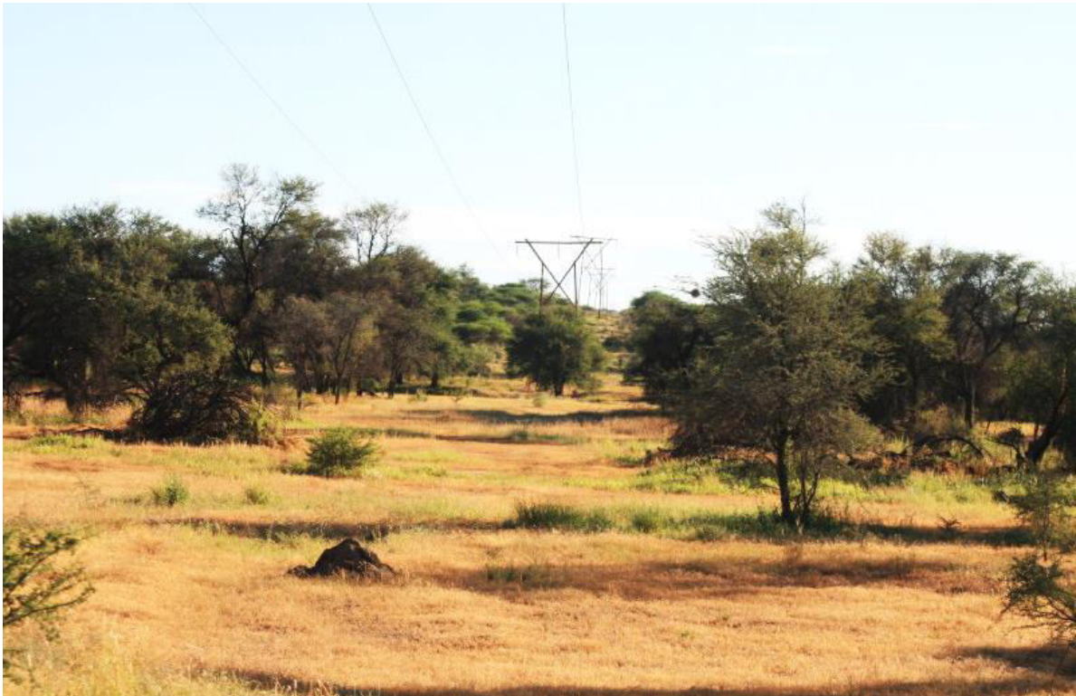
Figure 2. The larger well vegetated ephemeral drainage lines along the route are viewed as a sensitive habitat (“high”).
