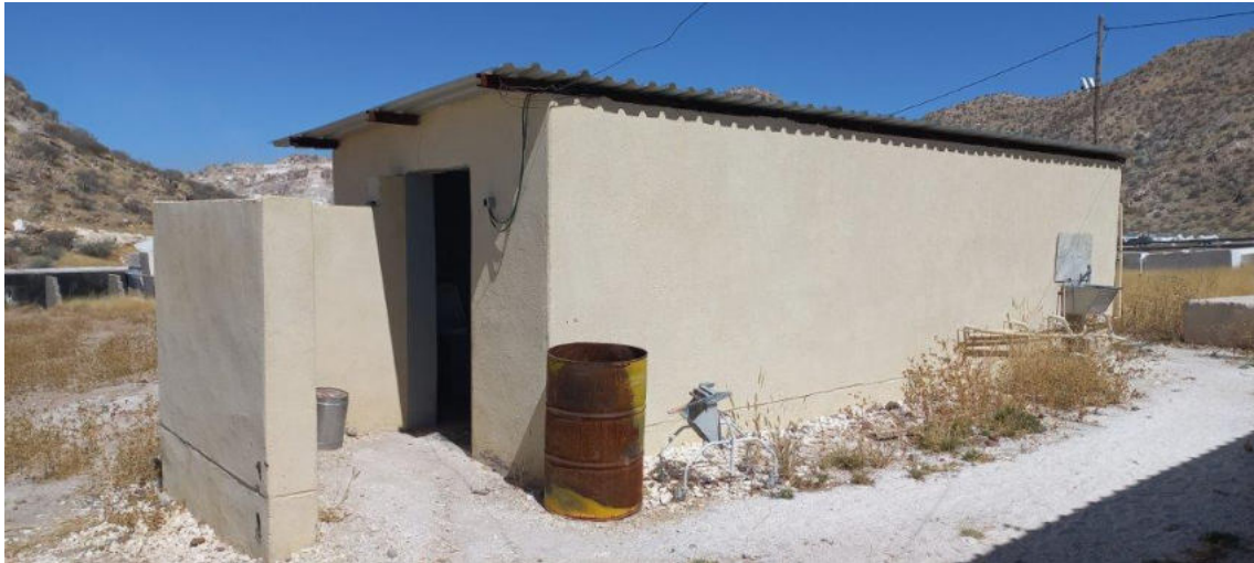
Photo 22 – View of ablutions on-site, well kept, tidy and neat.
