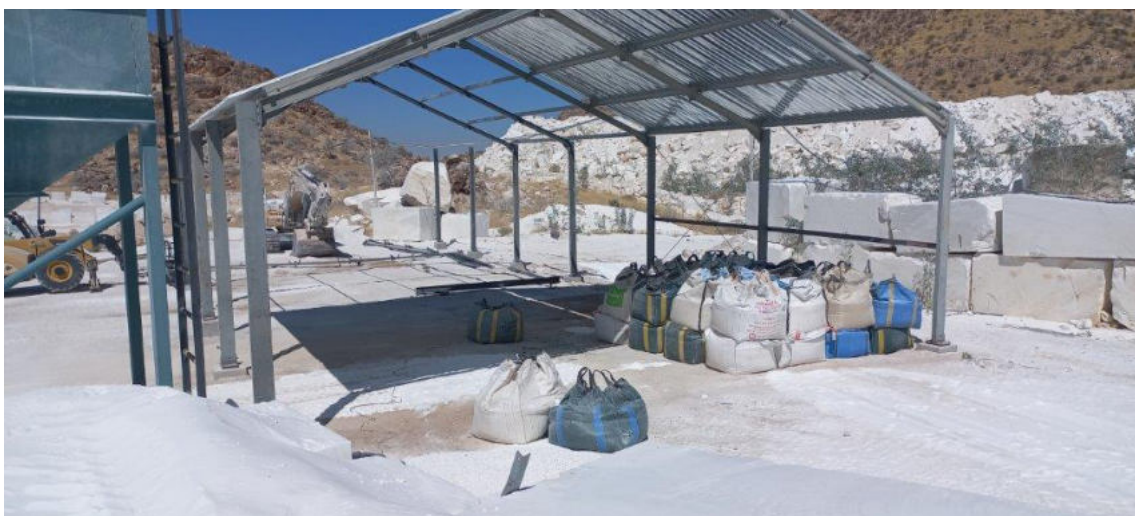
Photo 15 – View of under roof storage area.
