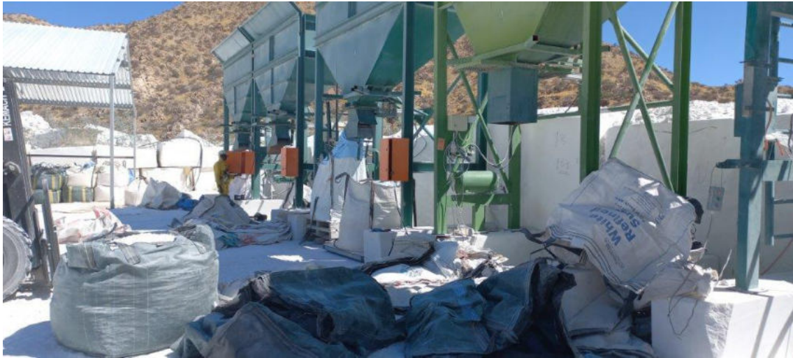
Photo 16 – View of stone bagging section.
