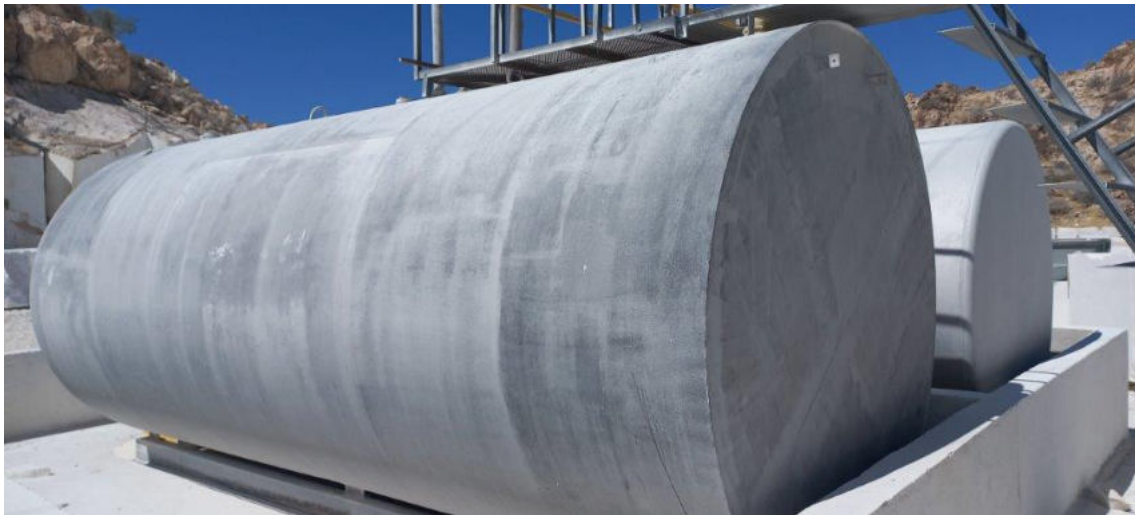
Photo 17 – View of fuelling area, well maintained.
