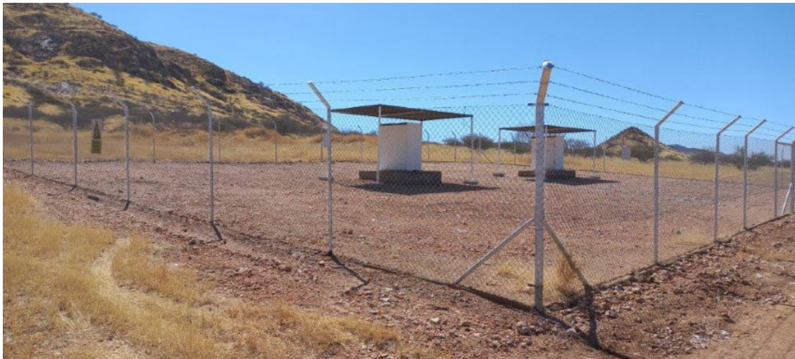
Photo 26 – View of dynamite store area, well maintained and kept safe.
