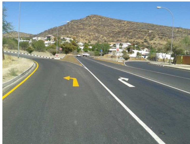
Figure 16 | B6 Road before the intersection with Sam Nujoma Drive
