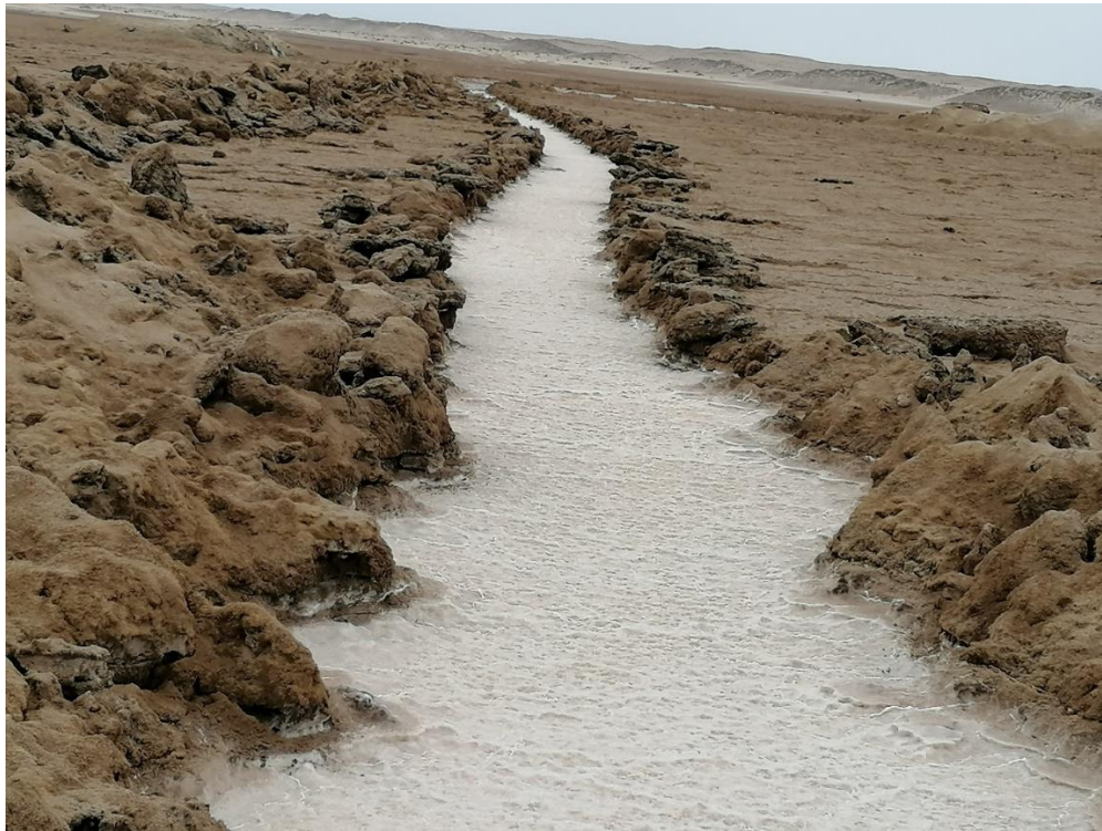
Figure 2: Shows a channel made to allow salt water to run to another man-made earth dam.
