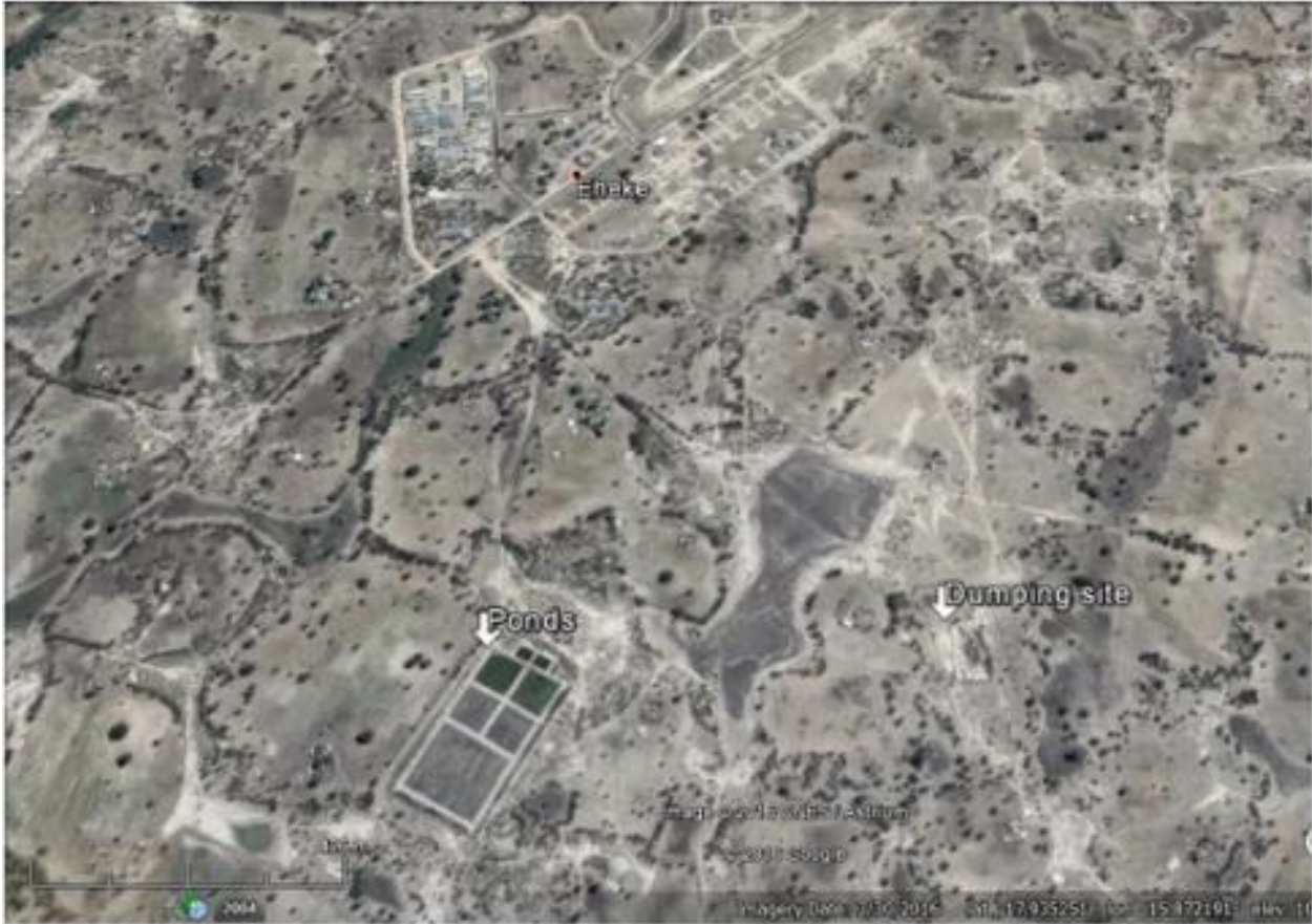
Aerial view of Ekeke Oxidation ponds
