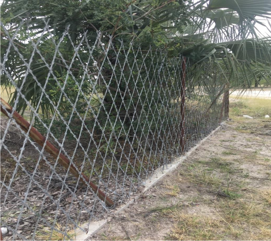
Figure 4 – Security fence around the perimeter of the oxidation ponds with trees to be trimmed
