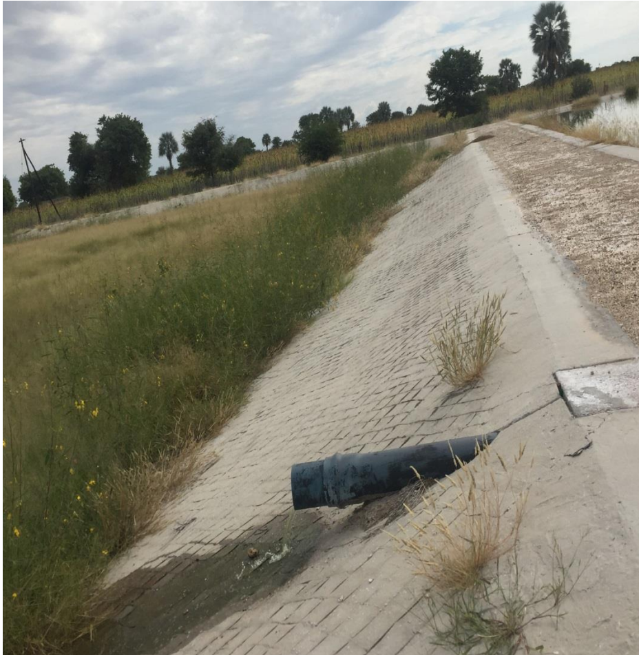
Figure 8– Slow flow into the evaporation pond - some vegetation to be removed
