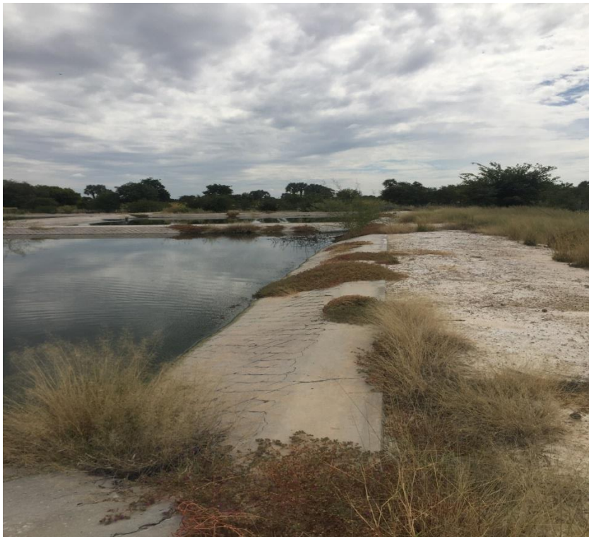
Figure 6 – Wastewater in anaerobic ponds– some vegetation to be removed
