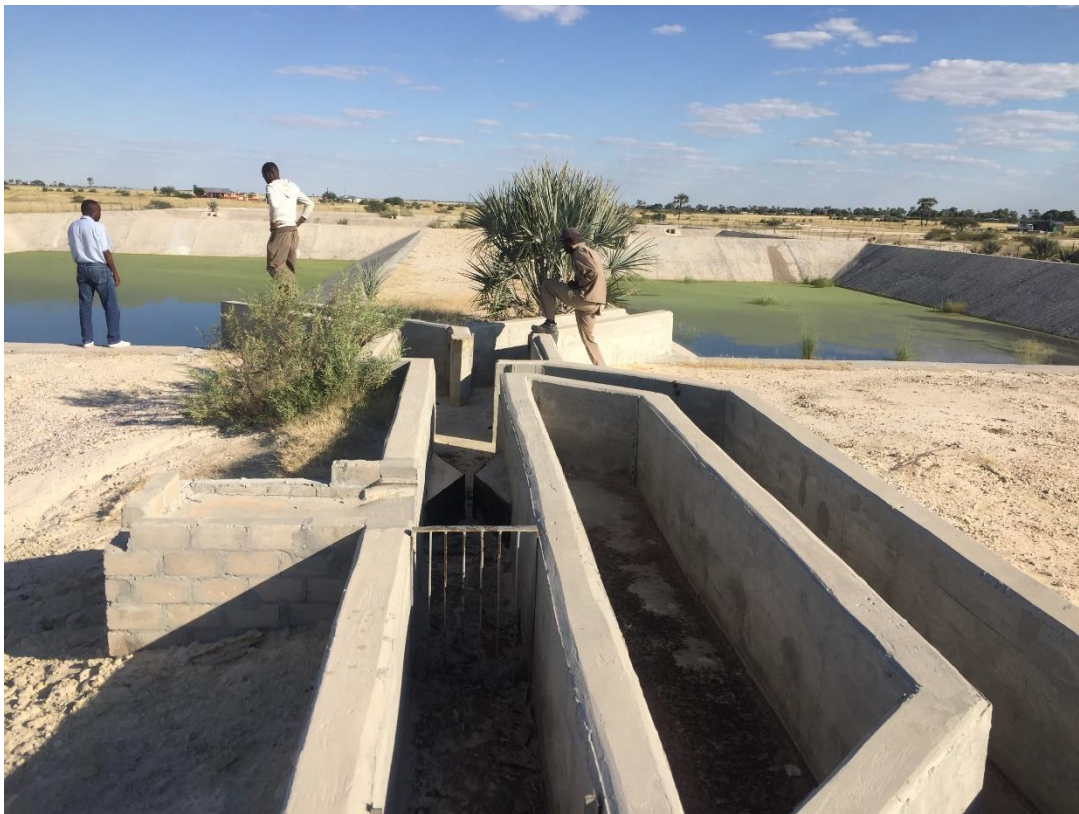
Figure 5 – Flow splitter installation and the two anaerobic ponds
