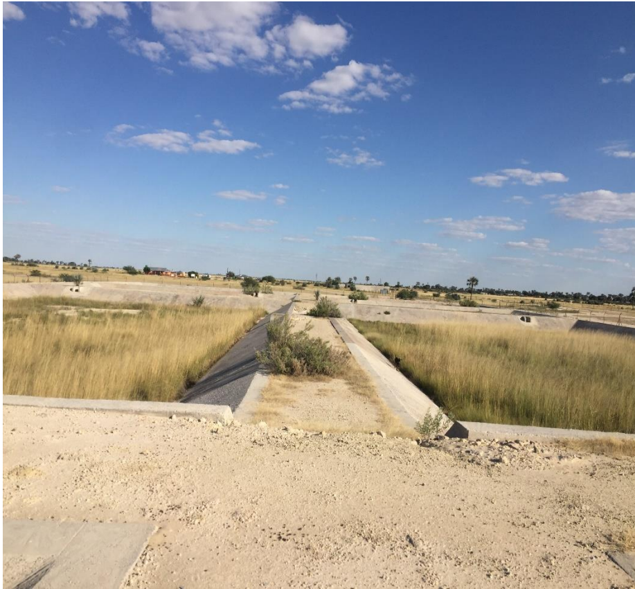
Figure 6 –Facultative Ponds with vegetation to be removed
