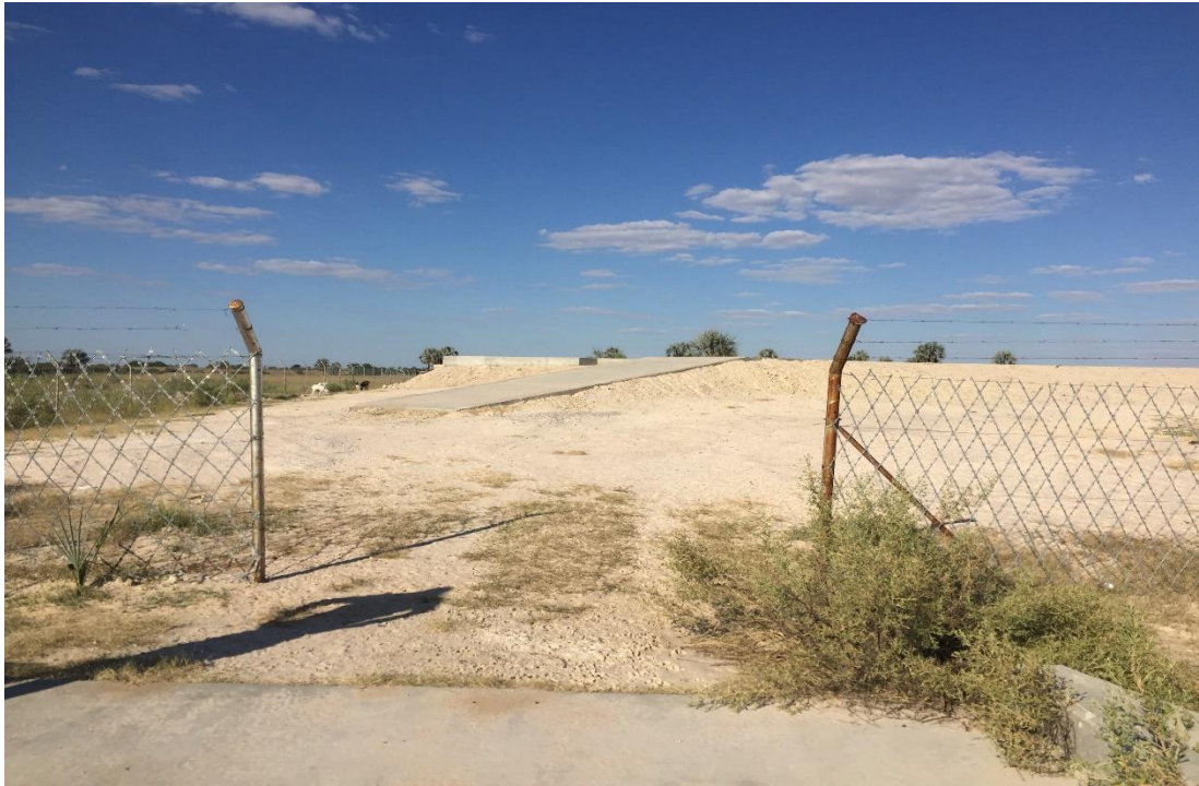
Figure 4 – Security fence around the perimeter of the oxidation pond site with missing gates
