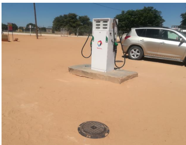
Photo 3. Existing pump and underground tank
