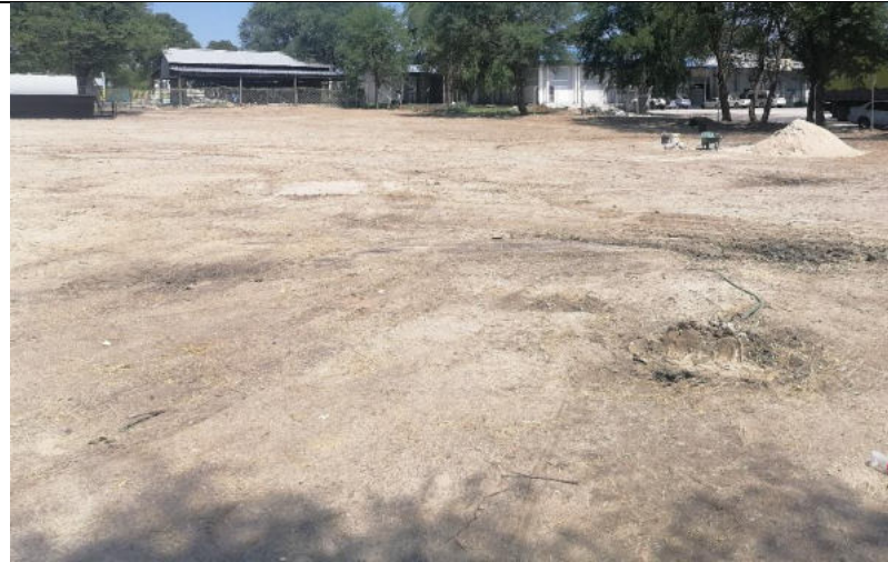
View of the site where storage tanks will be set up
