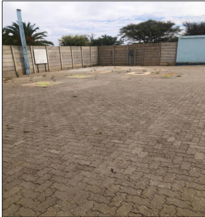
Figure 6: Fuel Station Courtyard – Fenced off.
