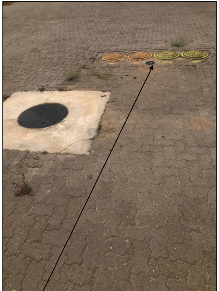
Figure 5: Underground Tanks – To be replaced.
