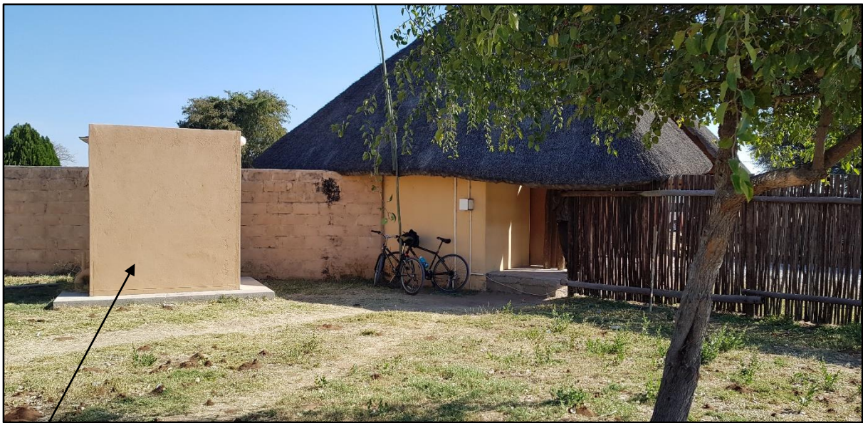
Figure 6: Added ablution facility for the Guardhouse
