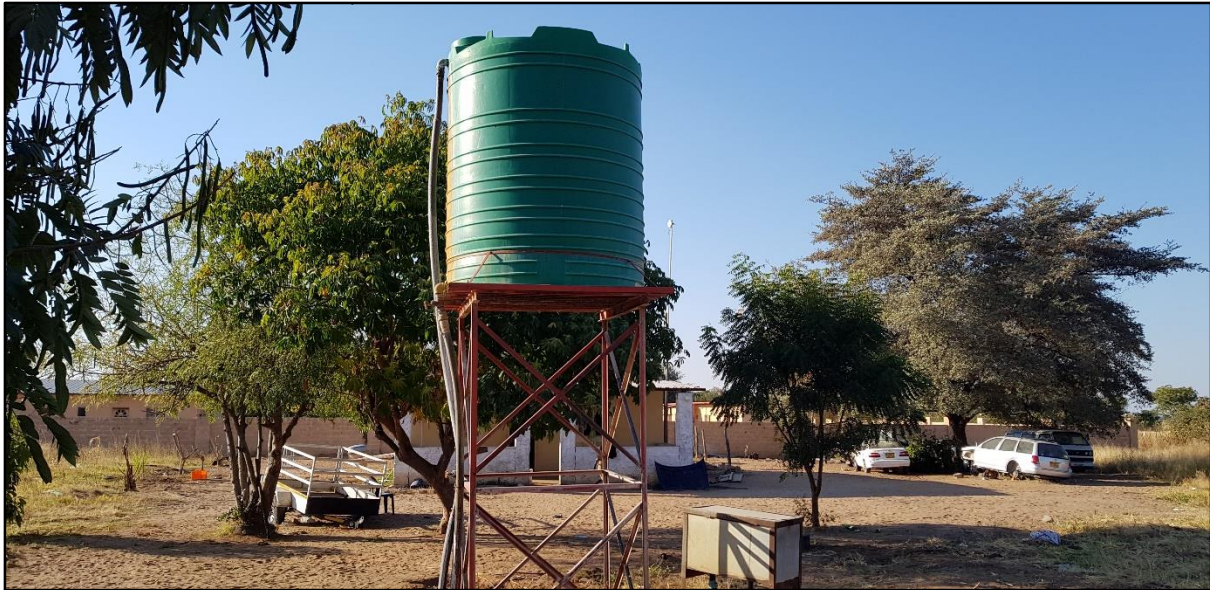
Figure 4: Borehole used by the community
