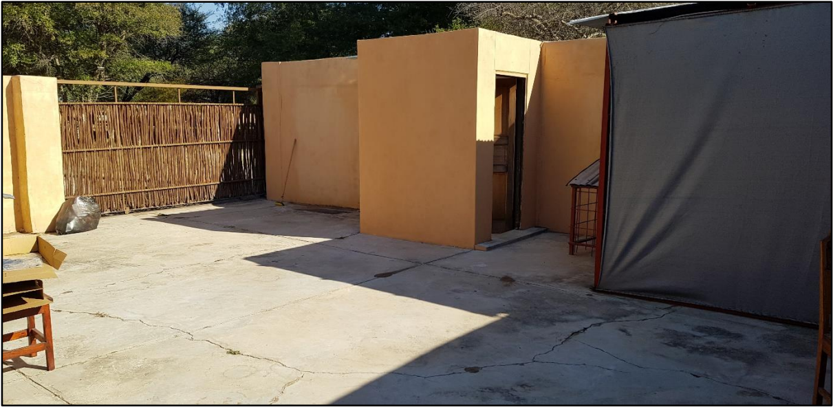
Figure 7: Added ablution facility for the kitchen staff
