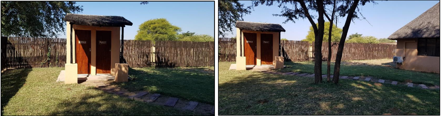
Figure 5: Added ablution facilities for the conference hall
