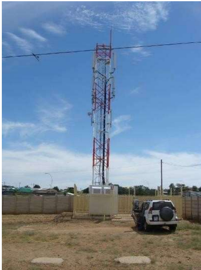
Figure 2-1: A typical red and white painted lattice tower structure
