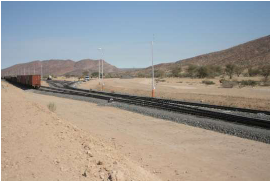
Figure 5-9: The well vegetated Aroab River, a tributary of the Khan River, in the Kranzberg Station area is visible in the background
