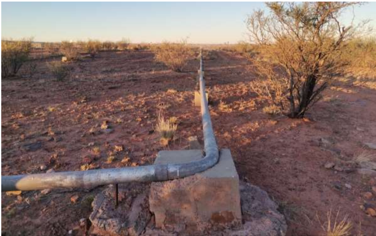
Figure 7: Existing above ground GMS pipeline
