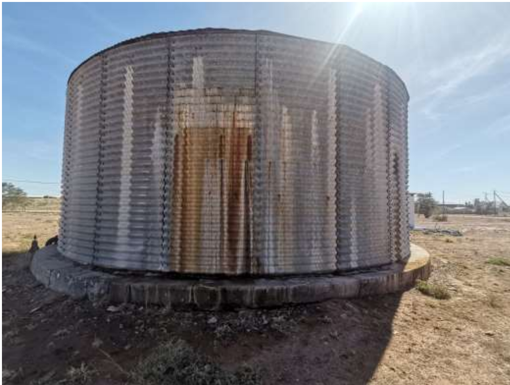
Figure 12: Existing ground level reservoir
