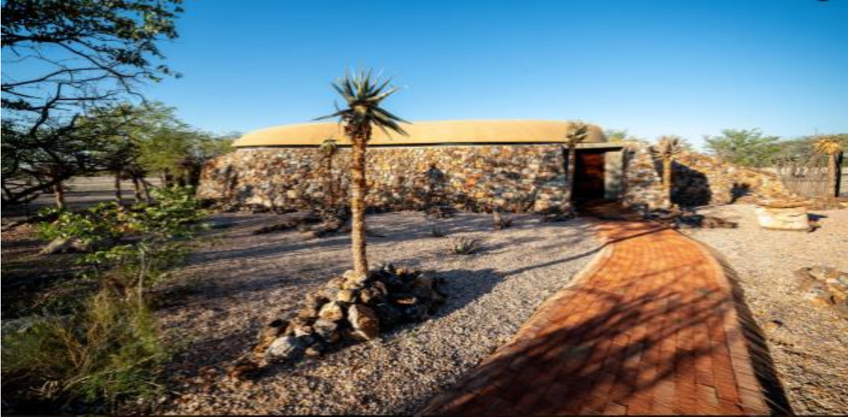
Figure 5. Exterior of a guest unit.
