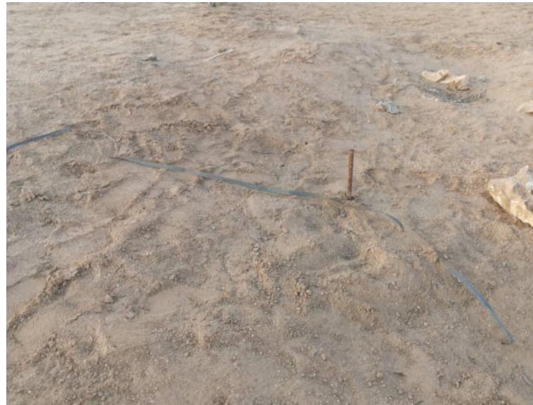
Surveying pegs and existing services on portion 127, Henties bay Townland No. 133
