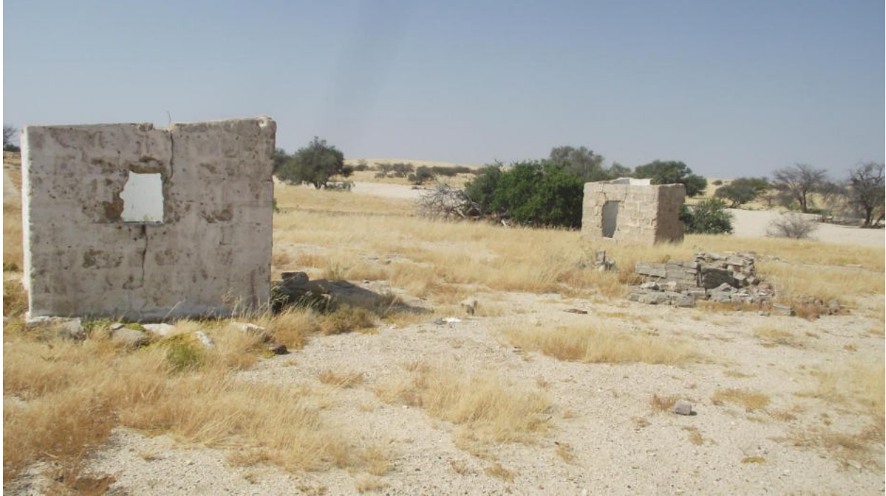
Figure 3: Ruined building structures on farm Goieie Geluk within EPL 8759 (Sources: Authors 2022).
