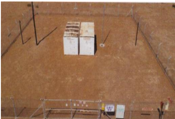
Photo 2. ANPP Warehouse ( illustrative )
