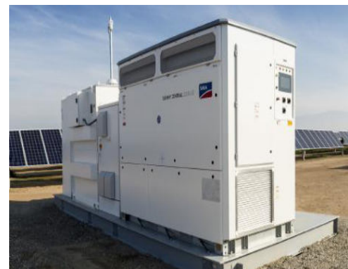
Figure 5: PV Panel Inverters
