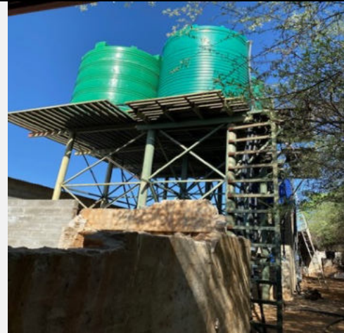
6 x 10000 L tanks filled with water from the river.
