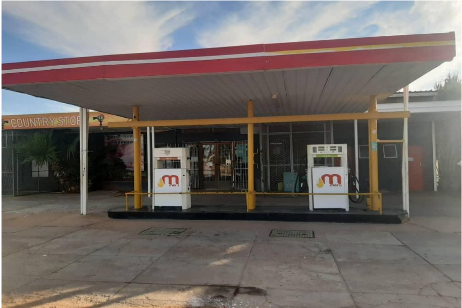
The filling in station
