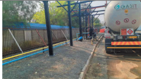
Photo 2-3 Gantry for offloading LPG
