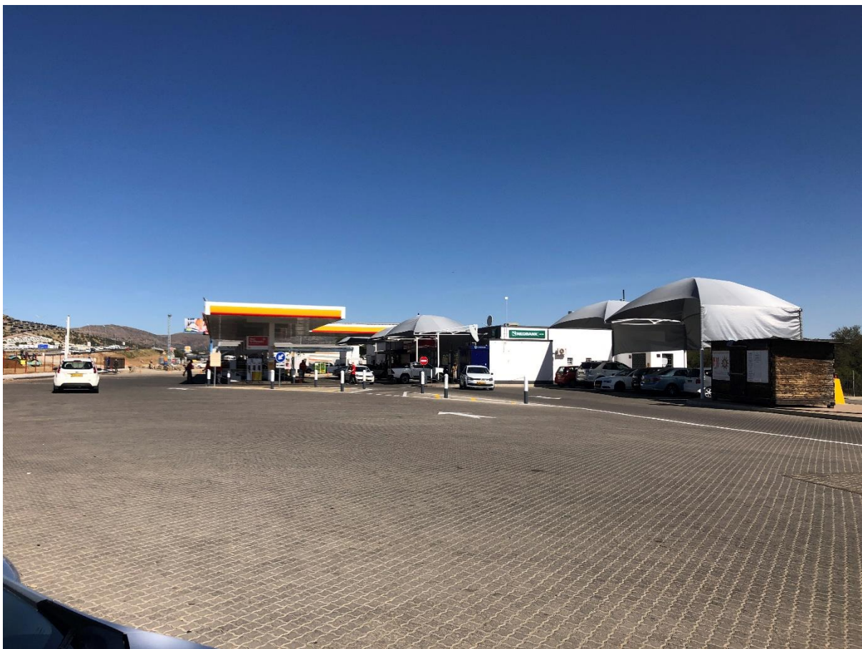
Figure 4 Image of the current fuel station set up.
