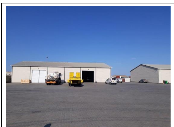
Photo 5. South western view from installation location
