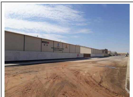
Photo 3. Alternative site access / exit in Gamberg Avenue
