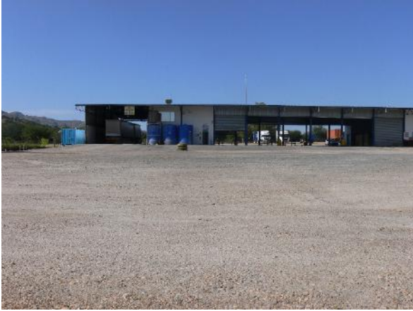
Photo. 3.2.3 Warehouse with wash bay, offices and workshop on the left
