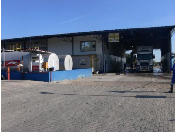
Photo. 3.4.1 Wash bay and filling station
