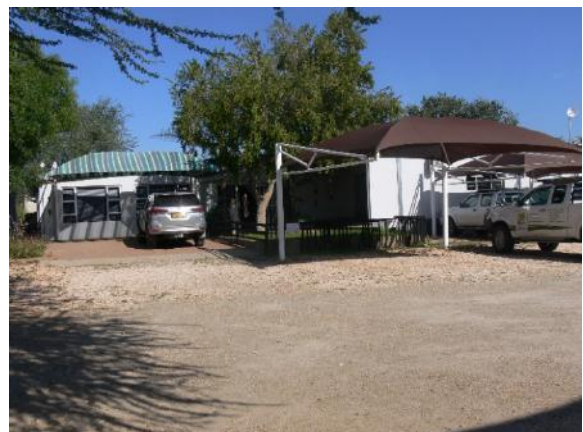
Photo. 3.2.2 Offices on Portion 18
