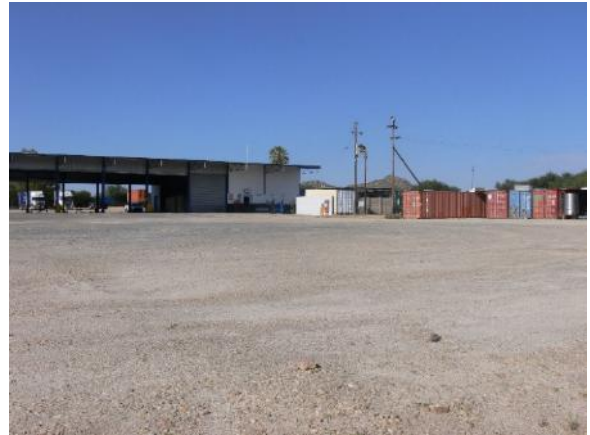
Photo. 3.2.4 Warehouse with workshop and storage containers to the right
