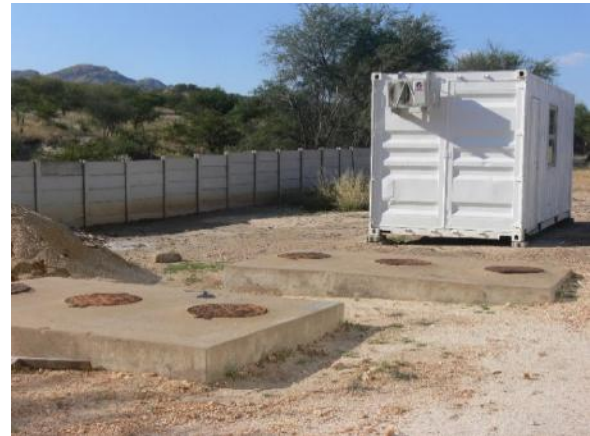
Photo. 3.3.8 Ablution and septic tank Portion 22
