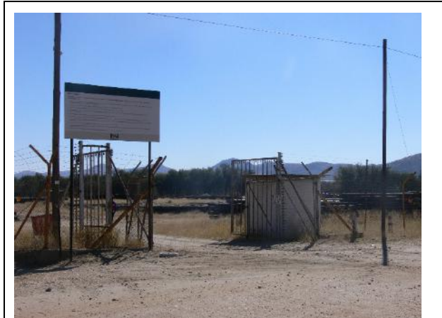
Photo 3.5.3 NamPower open camp storage facility bordering the Project Site
