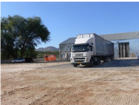
Photo. 3.2.7 Cerebos salt factory (viewed from the north)
