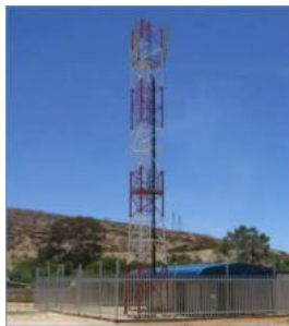
Figure 1: Example of Lattice Network Tower erected by PowerCom
