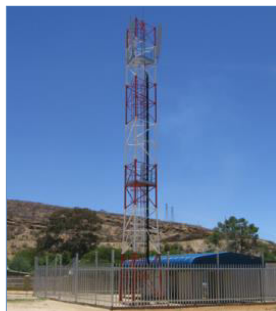
Figure 2: Example of the Lattice Tower ( https://powercom.na/ )
