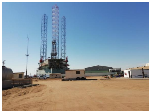
Photo 3. Northern view from project location
