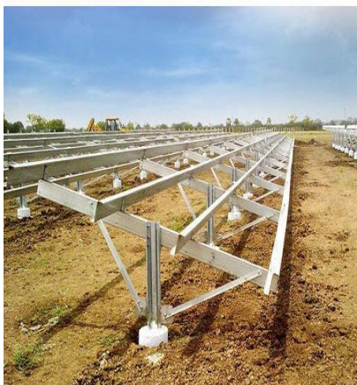
Figure 3: Completed PV Panel Mounting
